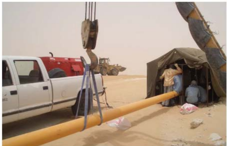
Oil pipeline construction
