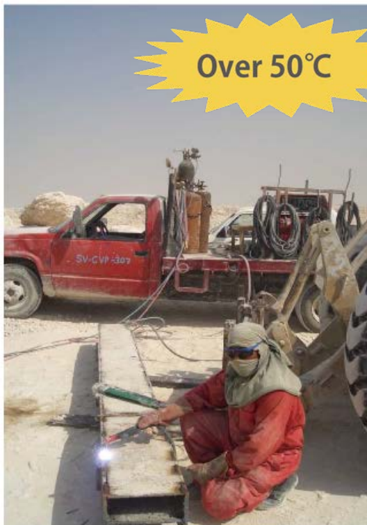
Maintenance of construction machinery
